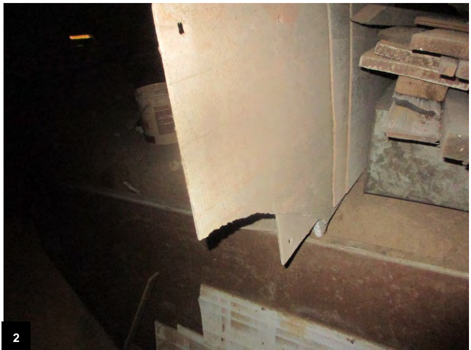
Sample 8 – Concrete Panels in Basement– 15% Chrysotile
