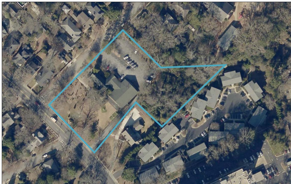
Aerial view of subject property at 465 Clairemont Avenue. Source: DeKalb County Imagery 2022.
