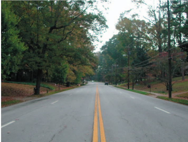
Top: West Ponce de Leon Avenue at its western portion conforming to the Section recommendation (Figure III.10).
