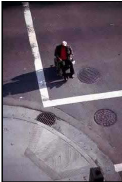
Figure 1. Poorly designed curb ramp forces individual into the intersection (from PBIC Image Library, Dan Burden)
