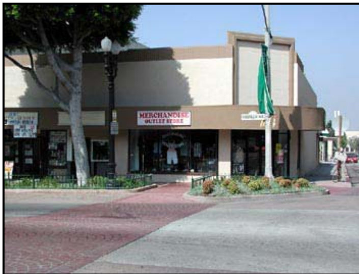
Figure 2. Well defined curb extension, perpendicular curb ramps and crosswalks set back from intersection (from PBIC Image Library, Dan Burden)
