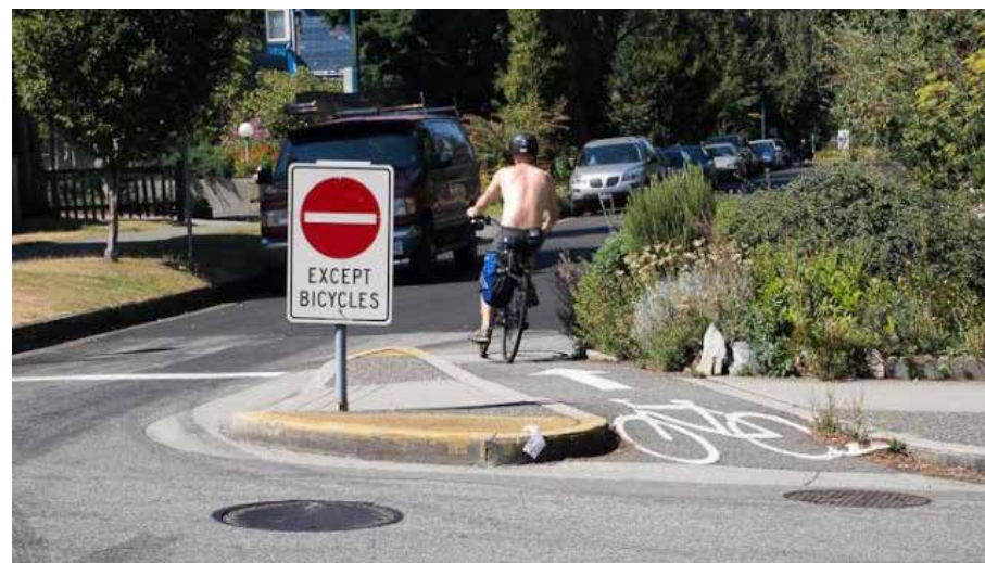
Neighborhood Greenway example showing limiting vehicle entry while utilizing signage and pavement markings for cyclists.
