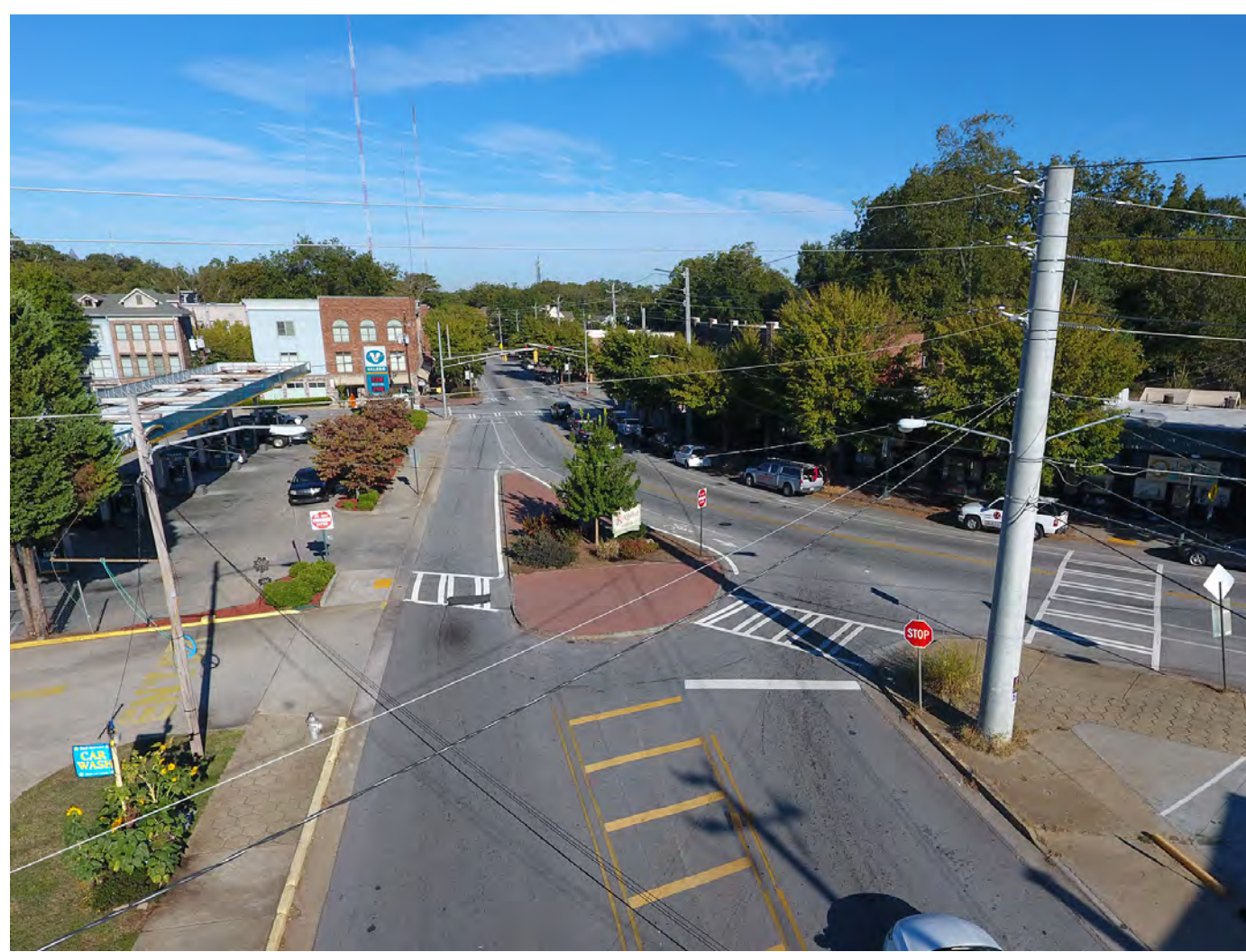
① Oakview Road and Hosea Williams - Transition
