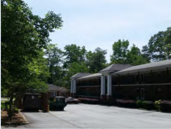
Existing Conditions at 1111 Oakview Rd.
