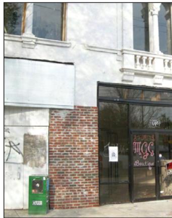
Inappropriate: The materials used in alteration should always be “in-kind,” so that they appear to be what is historic to the structure. Materials such as this brick on a stuccoed façade should never be seen.
