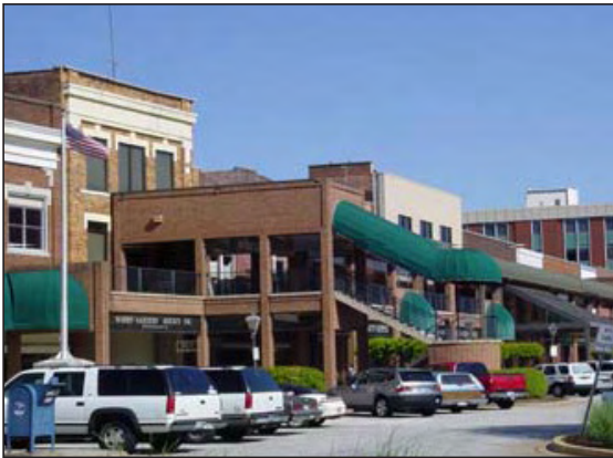
An inappropriately designed addition that obscures the historic building is not allowed.
