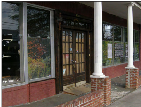
Replacing commercial doors with residential style doors or doors inappropriate to the time period of the building should not be done.
