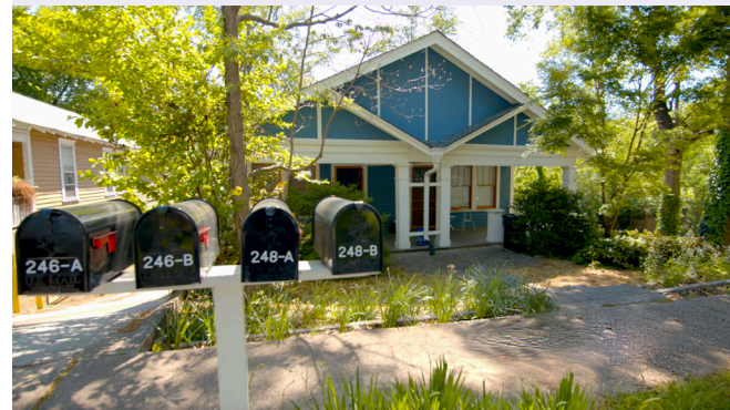
Renovated quadplex, Decatur, Georgia
