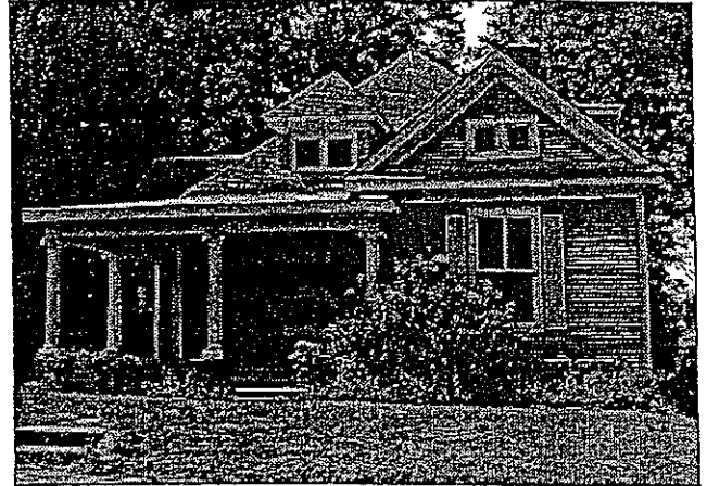
The asymmetrical massing and Ionic order columns identify this house as Colonial Revival.
