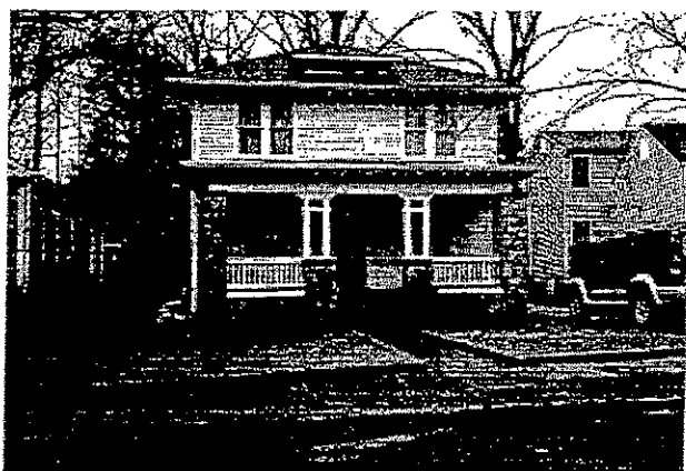
Porches are critical architectural elements subject to full exposure to the elements.
