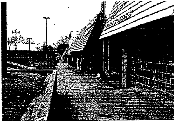
Adding false fronts and pent roofs is not recommended.
