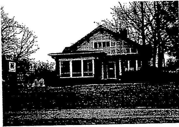
A good example of enclosing the front porch of a residential building, reused for business.
