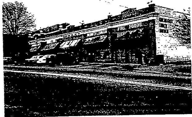
Neighborhood commercial 'storefront' building on West College Avenue.
