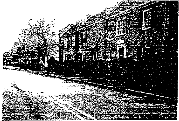
Townhouse development in the transitional belt should be sited close to the sidewalk.
