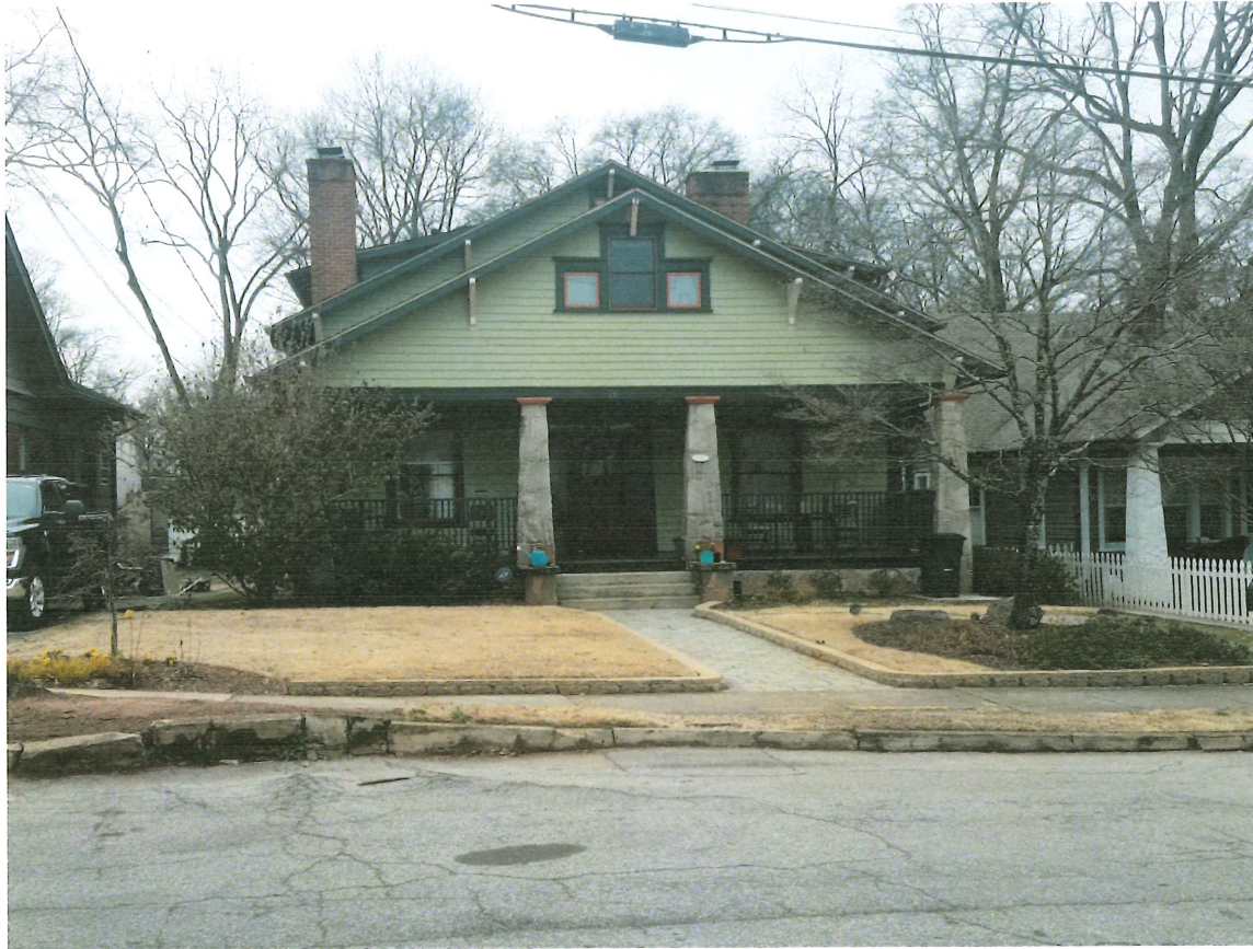
Front Elevation - 131 Kings Hwy (neighboring property)
