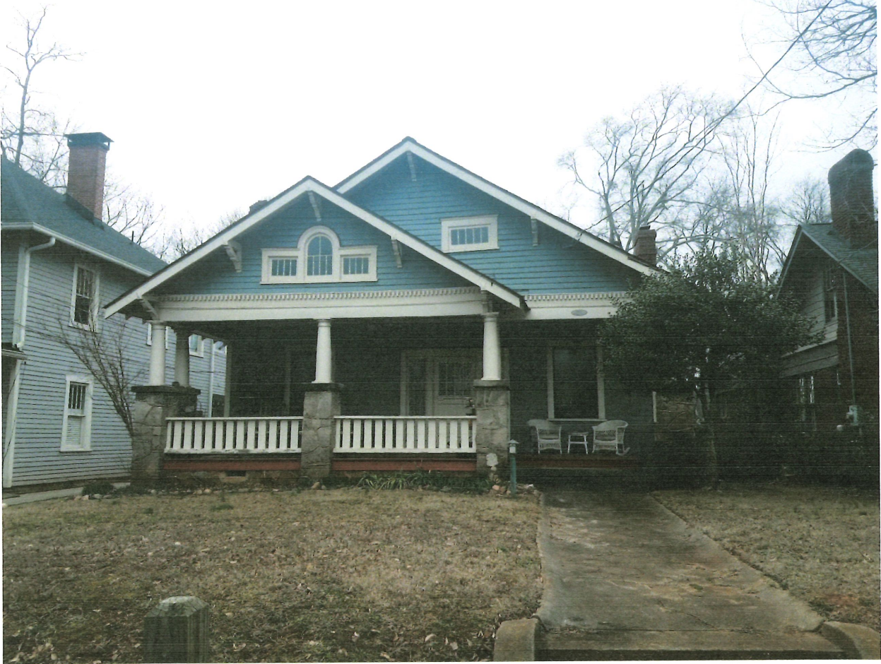
Front Elevation - 139 Kings Hwy (neighboring property)
