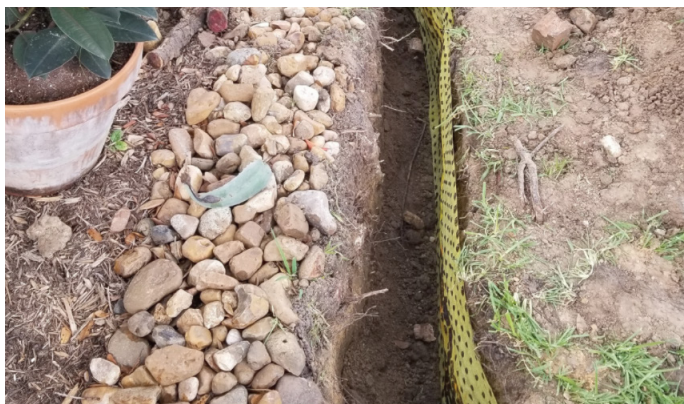
Modified French Drain Installation Source: crackedslab.com
