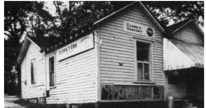
Clark's Grocery, operated by Archie Clark and his wife, Dovie, provided first-class service to African-American residents of Decatur from the 1930s until 1978. On the back side, facing White Street, was a shoe store and dry cleaners.
