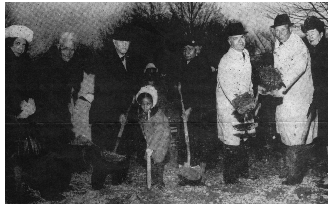
Groundbreaking for the new Antioch AME Church on Hibernia Avenue in 1965. The church stood for 90 years on the site of the recently demolished Callaway Building, across Trinity Place from the DeKalb County Courthouse. The Hibernia Avenue church was bulldozed to permit construction of the Swanton Heights neighborhood.
