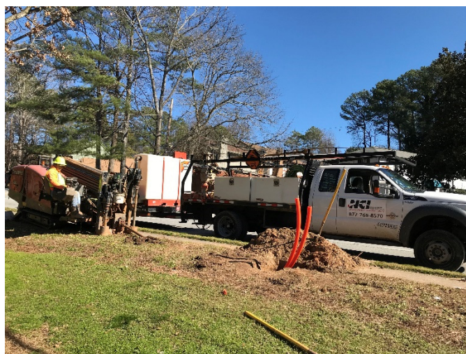
Fiber ring installation
