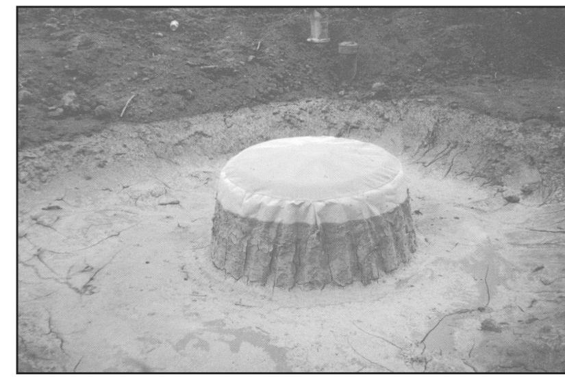
Figure 6-28.7 Equivalent Inlet Sediment Trap
